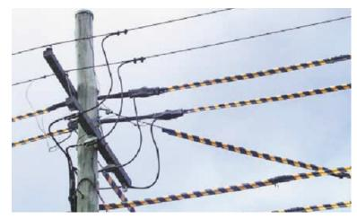
Figure 16 – Tiger tails fitted to overhead power lines
