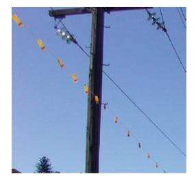
Figure 7: Illustration of a visual tape bunting fitted under overhead power lines.
