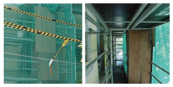
Figure 11 – Enclosure of overhead powerlines
