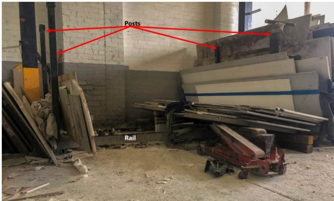
The post frame racking where the incident occurred
