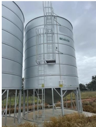
Access ladder to top of silo
