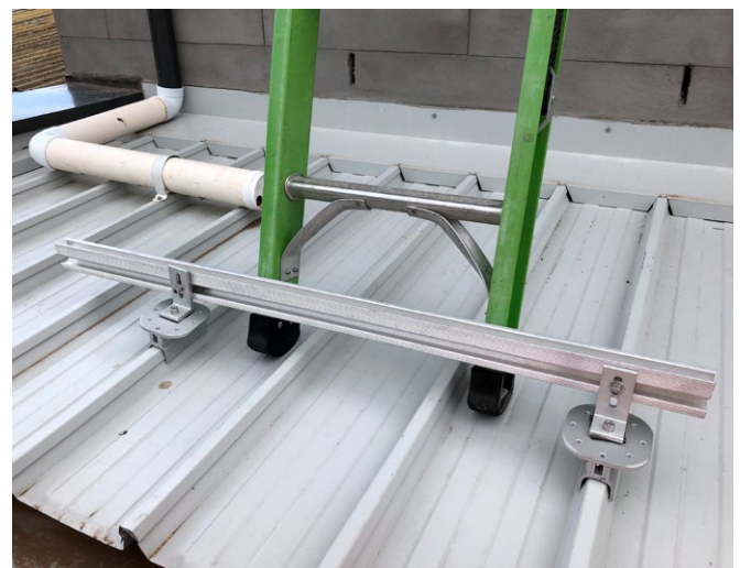
Image 2: Base of ladder secured on lower level roof
