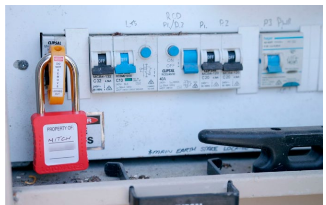
Image 11: Example of main electrical switch with lock
