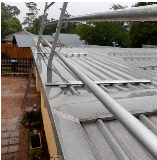
Images 3-6: Examples of temporary edge protection
