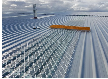
Images 8-10: Examples of physical barriers to manage risks of falling through skylights and brittle roof material.
