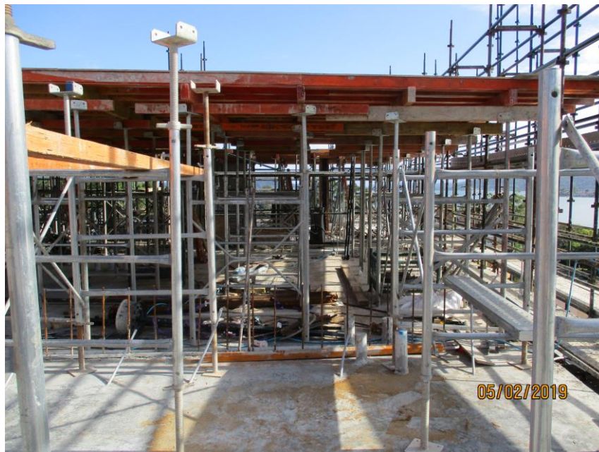
Image 1 – Construction site where work was being done.
