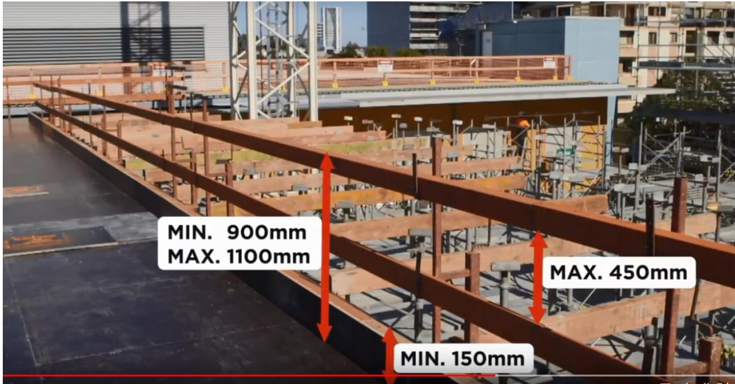
Figure 7 – Guardrails for prevention of falls
