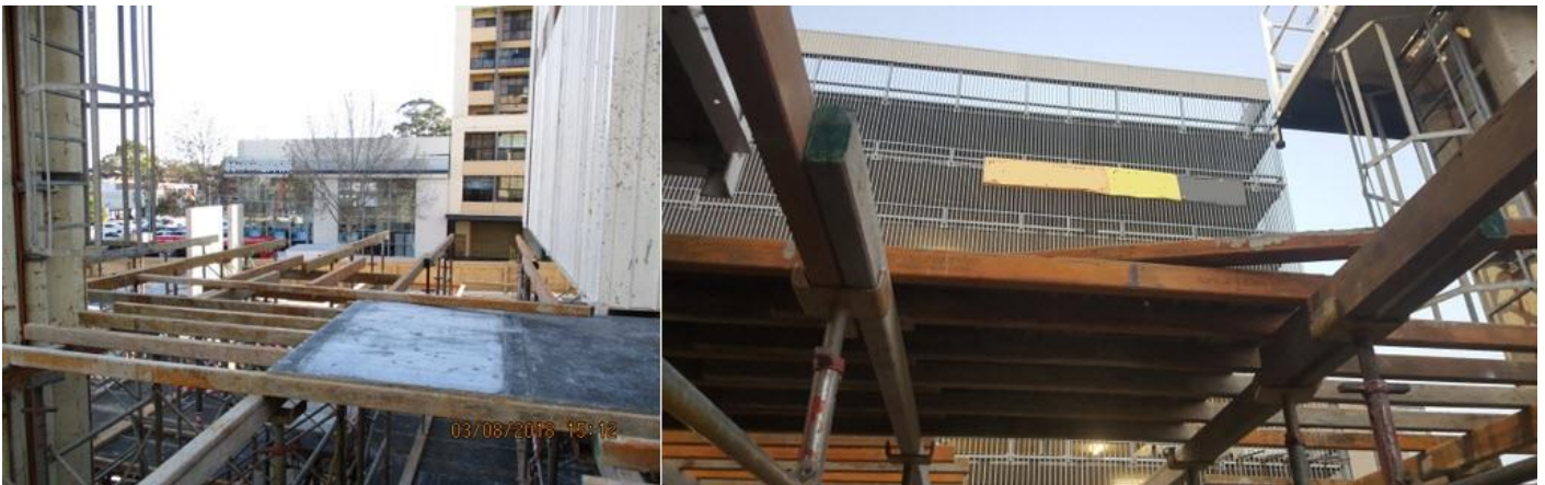
View of the formwork from the side and the level below.
