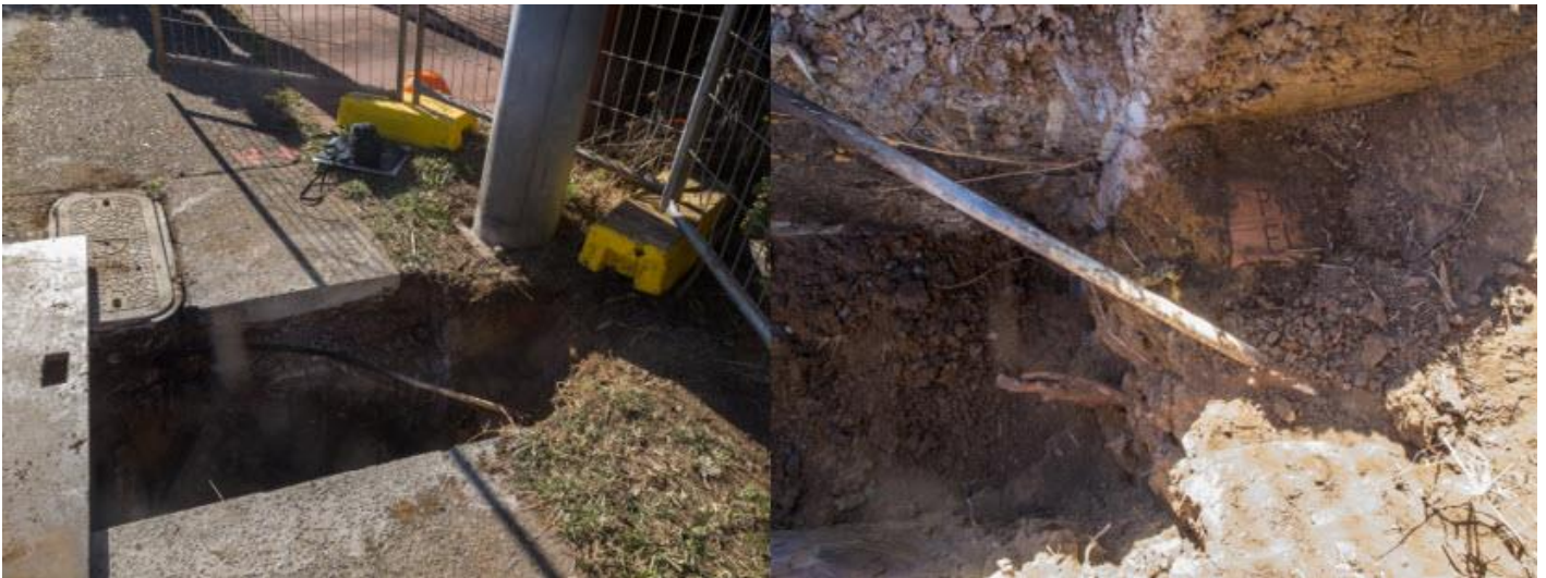
Photographs: Trench excavation site where works were being undertaken.
