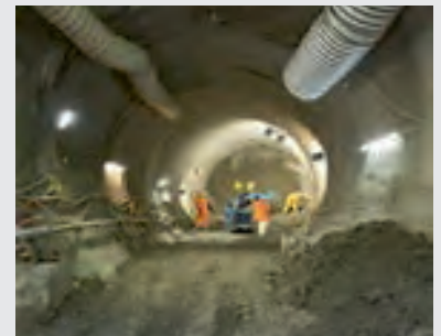
Tunnelling with ventilation
