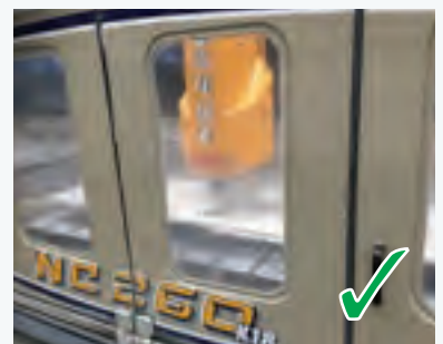
Water suppression for cutting
