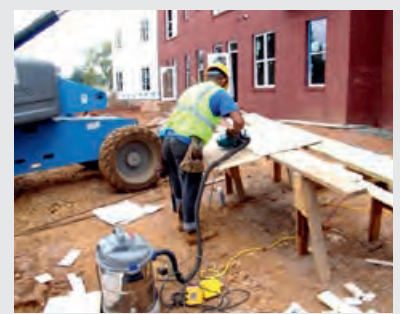
Cutting fibre cement sheet with dust extraction
