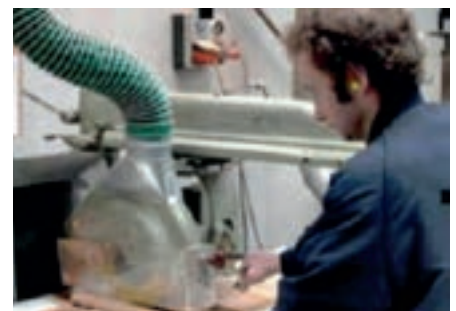
Local exhaust ventilation system attached to the saw
