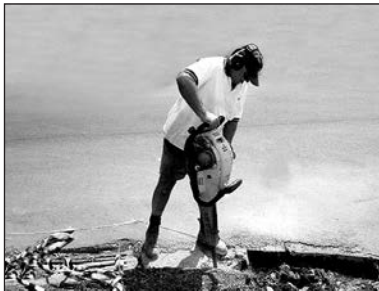
Operating petrol-powered jack hammer
