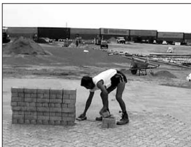
Laying paving blocks
