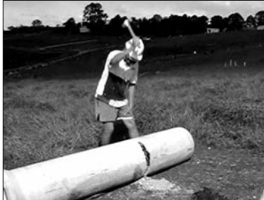
Cutting concrete pipe with hammer
