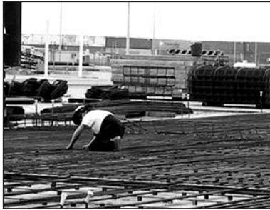
Steel fixing
