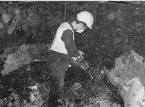
Figure 1: Worker using jackhammer to break up slag inside furnace
