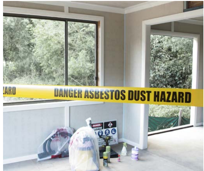
Asbestos hazard tape around removal area
