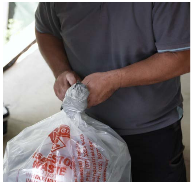
Goose necking asbestos waste for disposal at a site authorised to accept asbestos
