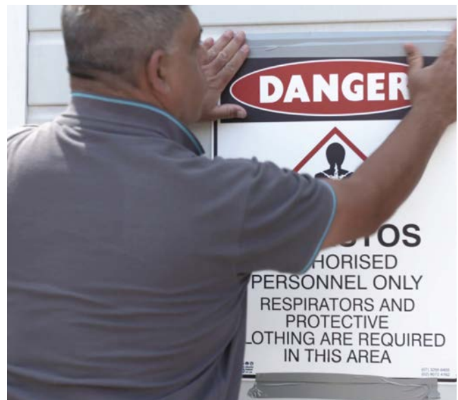
Putting up asbestos warning signs prior to removal
