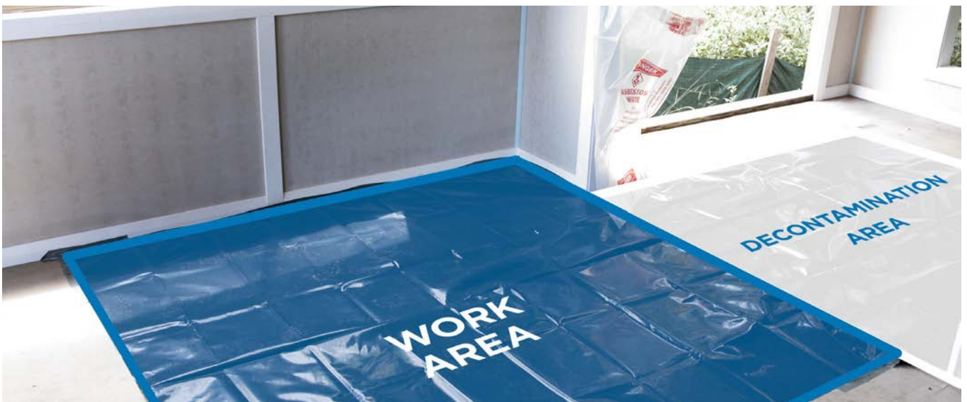
Asbestos Work area set up adjacent to decontamination area
