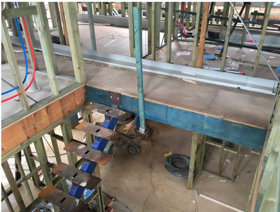
Image: View of the stair void and access stairs.
