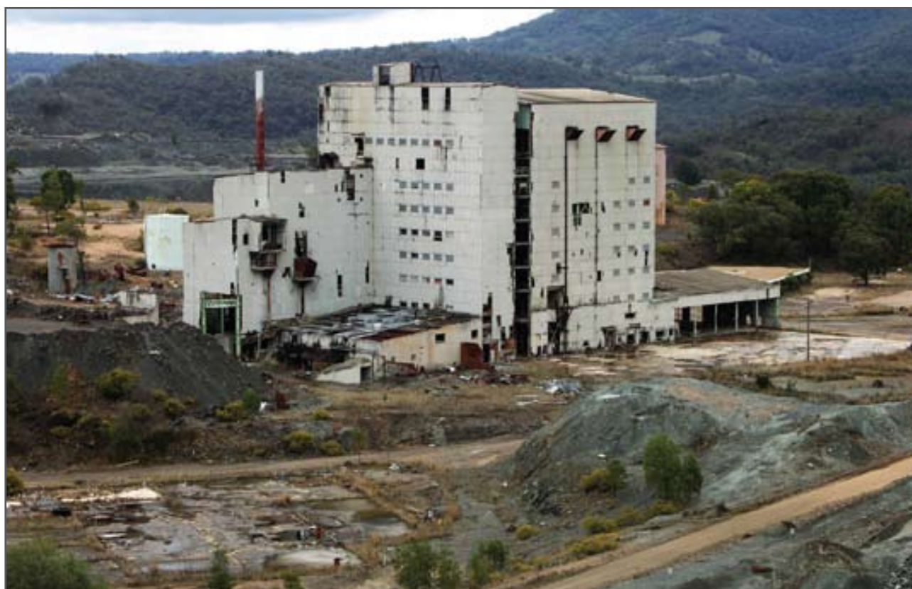
Photo 1. Abandoned mill house.
