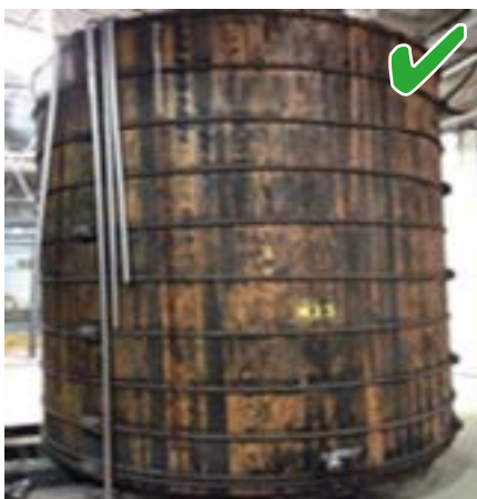
Photograph shows example of modifications made to large wood tank by installation of a test tap near base.
