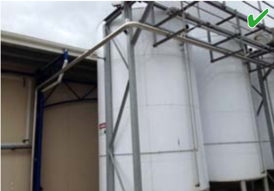
Retrofitting of overhead fixed lines helps to reduce trip hazards and improves efficiencies to enable manoeuvrability of other plant and equipment at this location.
