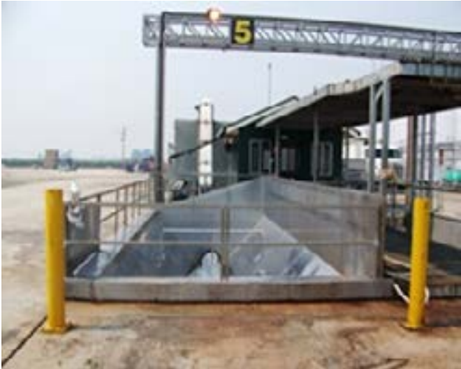
A fruit reception hopper with handrails and gate to prevent accidental falls into the auger area.
