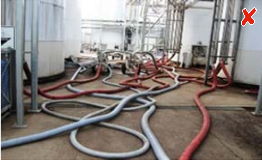
A result of poor organisation where hoses cause a trip hazard to workers involved in transferring/pumping operations.
