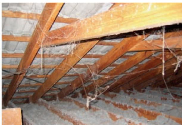
Loose-fill asbestos insulation inside ceiling space
